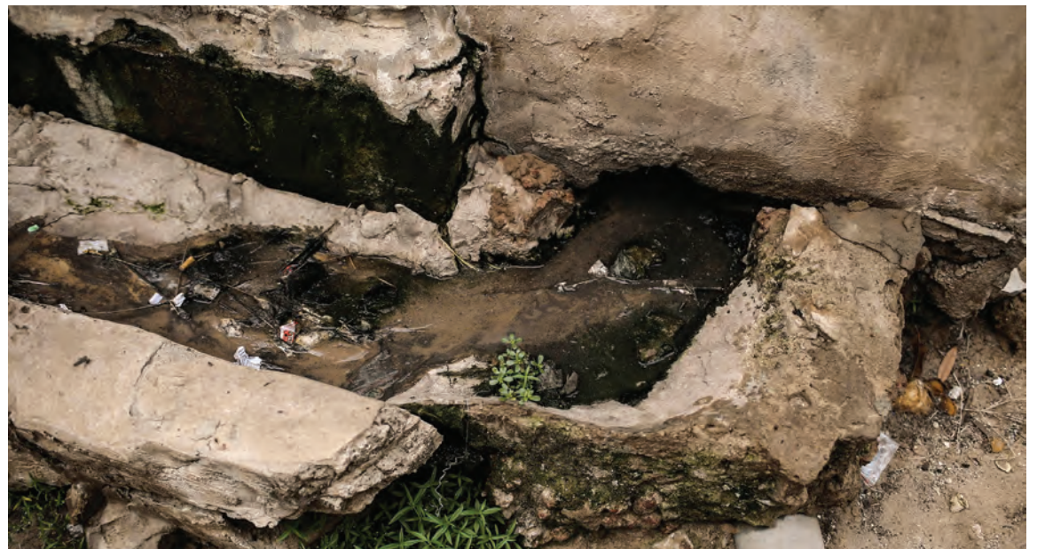
Mile 2, Central Prison, Banjul: A broken sewage pipe behind the latrines.
